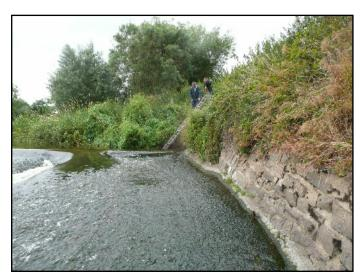
The weir is approximately 1.5 metres in height with a fish pass cut into the top of the weir on the right hand side creating a very strong flow of water across the face of the weir. At the base of the weir there is a gently sloping surface where a wide shallow slow moving wet interface exists between the bank and the rapid spillway.
