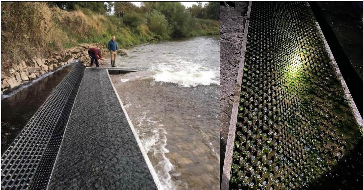
The pass now obstructs the natural migration route to the weir face.
