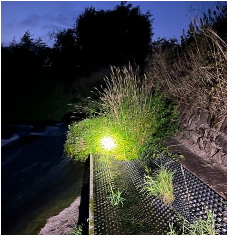
Pass dry blocked by vegetation
