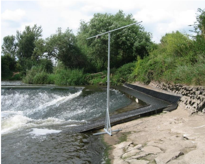
The pass now obstructs the natural migration route to the weir face.
