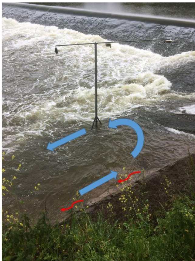
Mid flow conditions
