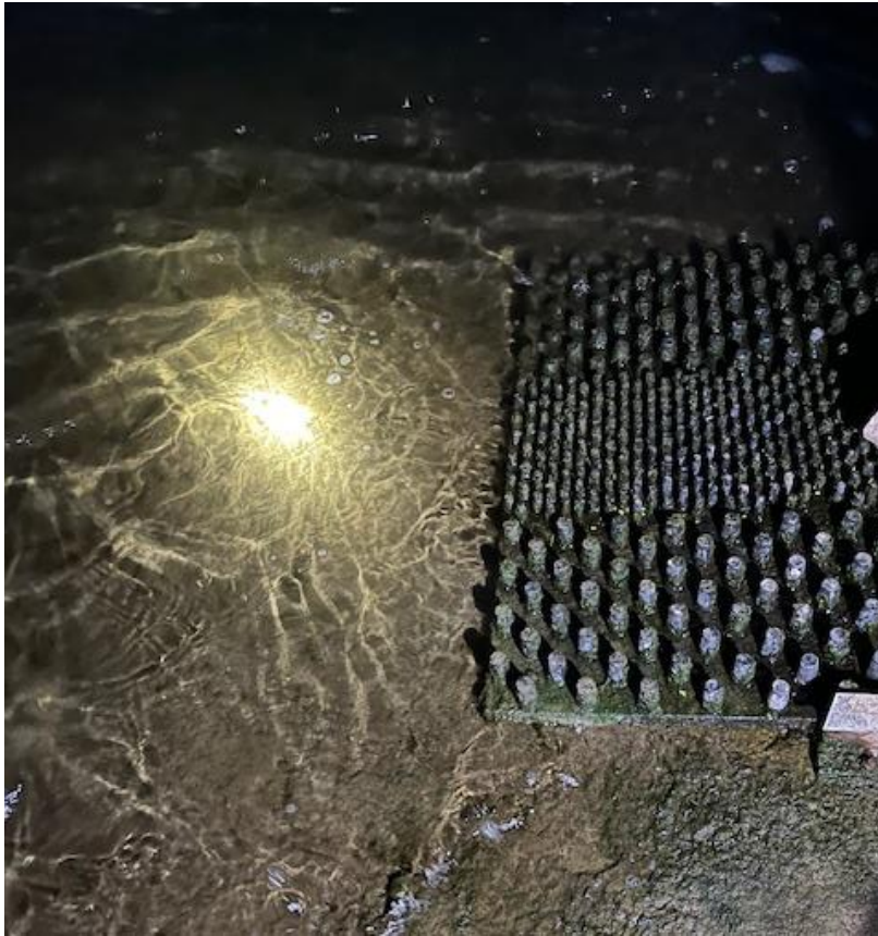
Dry Pass leader - No connectivity with river. Impassable.
