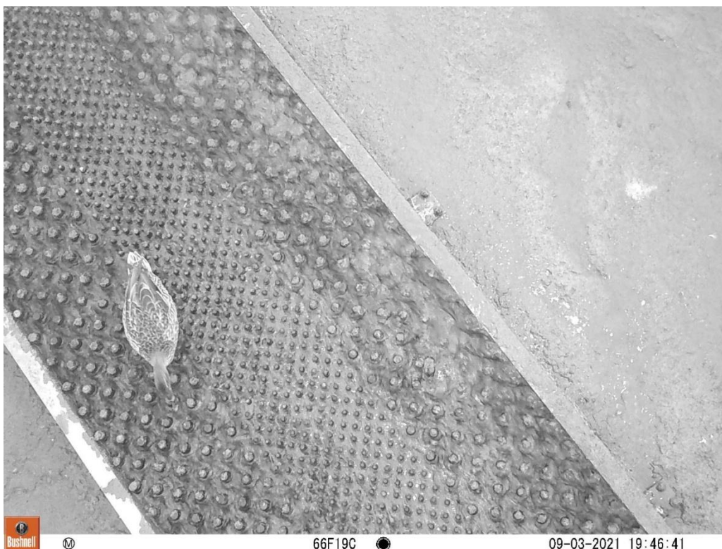
Pass with incorrectly installed substrate.
